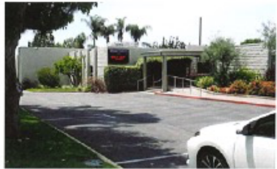
12 Secondary Campus Entrance
