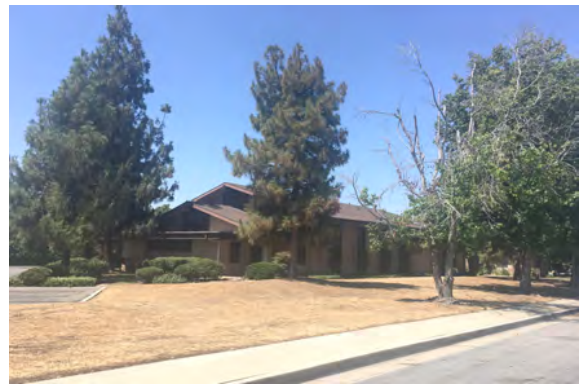
② Corner of Newport & Vanderlip Avenues looking southwest
