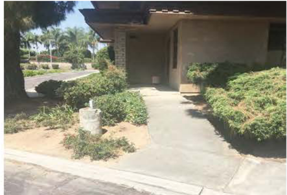
8 Rear of Sanctuary Walkway to be Removed looking west
