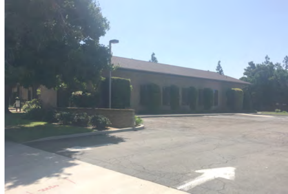
④ Vanderlip Avenue looking southeast at Sunday School
